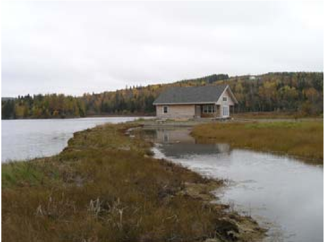
Figure 64. View of a new residence constructed in 2004 on the backbarrier beach ridges at Gillis Beach, Jamesville (Fig. 44, site 45). It is not known where the septic tank is located but it is obvious that the builder has not planned for increasing water levels as the narrow part of Gillis Beach is overtopped, eroded and flooded. The house sits on beach ridges built long ago when sea level was much lower (Photo R. Taylor, 27 October 2004).
