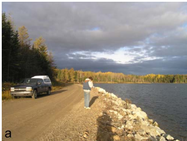
Figure 57: Many secondary roads such as this one (a) along North Basin are armoured by rock (PA290097; 29-October -2004) but are commonly less than 0.8 m above present water level (b).
